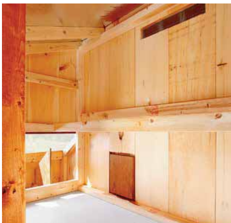
Interior view of L35 (page 71)
