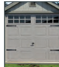
Carriage House Door with Windows
